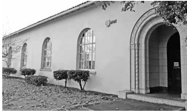
The building referenced by D.S. Smith in 1958 at Willow and Central still sports the AT&T logo and is owned by the company.
