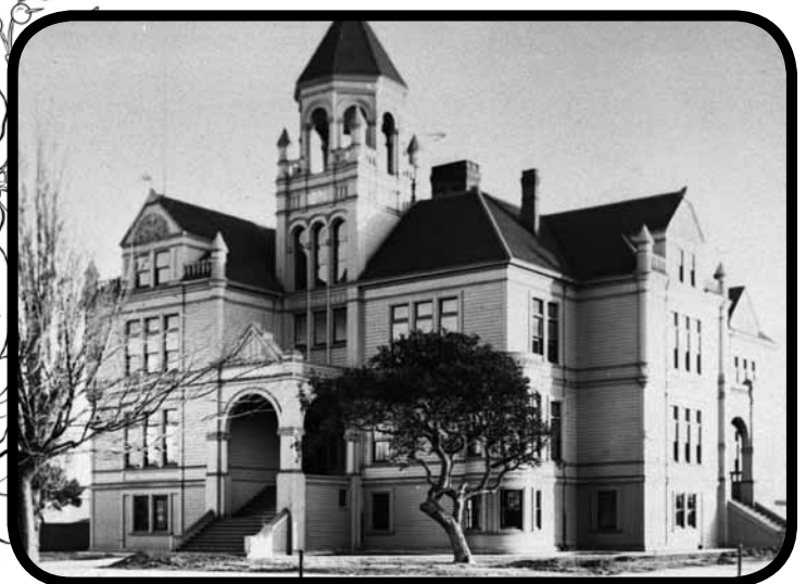
Longfellow School in the West End
